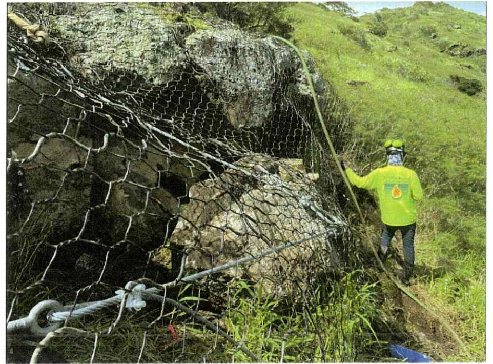
After: rock mitigation work in-progress
